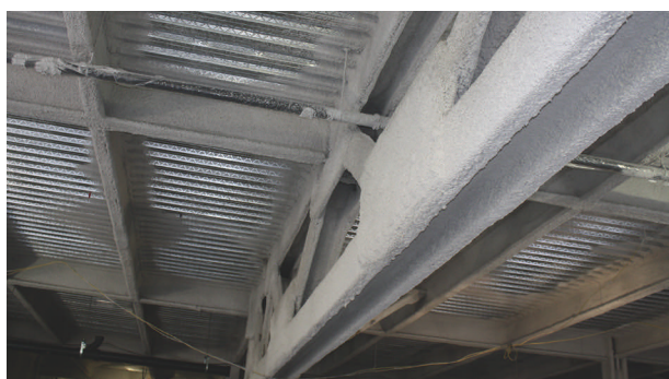
Figure 1: Steel framing with SFRM in place at Children’s Memorial Hospital under construction in Chicago. Inset shows the hospital’s signature handprint rendered in SFRM.
