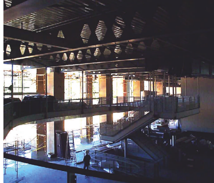
Left and above: The serpentine track in the Herrington Patriot Center is hung from the castellated steel roof beams used to accommodate the long span over the weight room.
