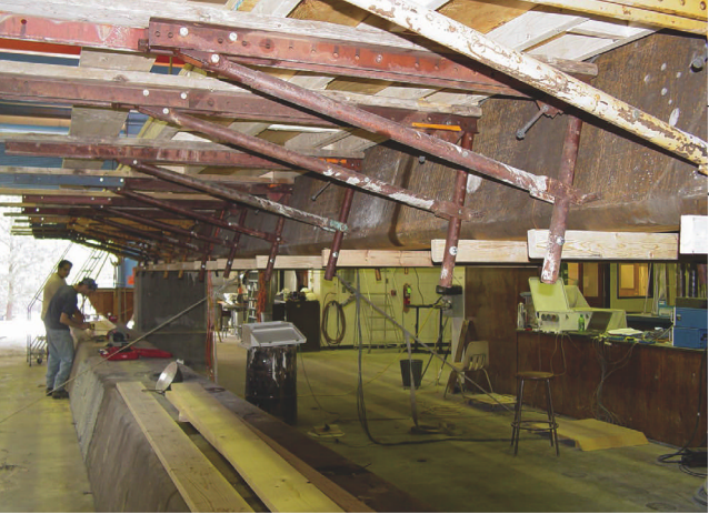
Fig. 2 Conventional forming materials and methods can be used to form the concrete deck on the folded plate girder.
