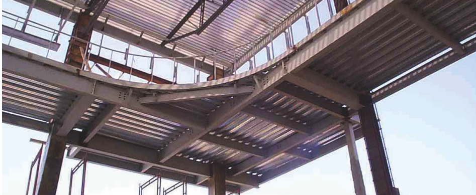
Above: Composite steel cantilevered running track in the Jerry D. Morris Recreation Center gymnasium is supported by composite steel columns.
