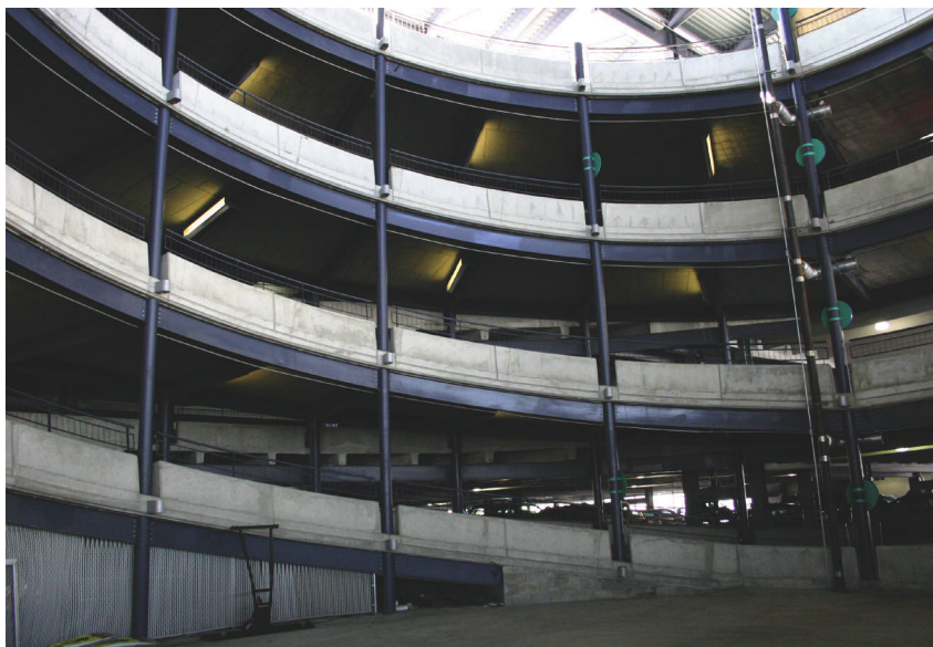
This page: The JetBlue garage at the Portland (Maine) International Jetport uses a steel framework on the spiral ramp to support the floor slabs.
